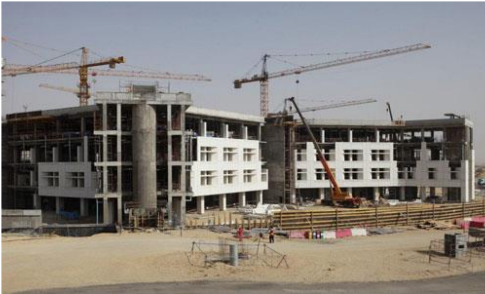
Figure 10: Progress on New KOC Hospital (14 th January, 2014)
