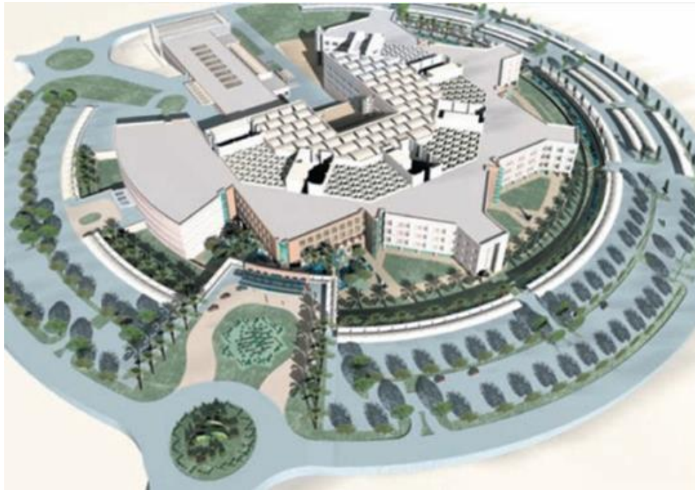
Figure 9: Schematic of New KOC Hospital Currently Under construction by Syed Hamid Behbehani & Sons
