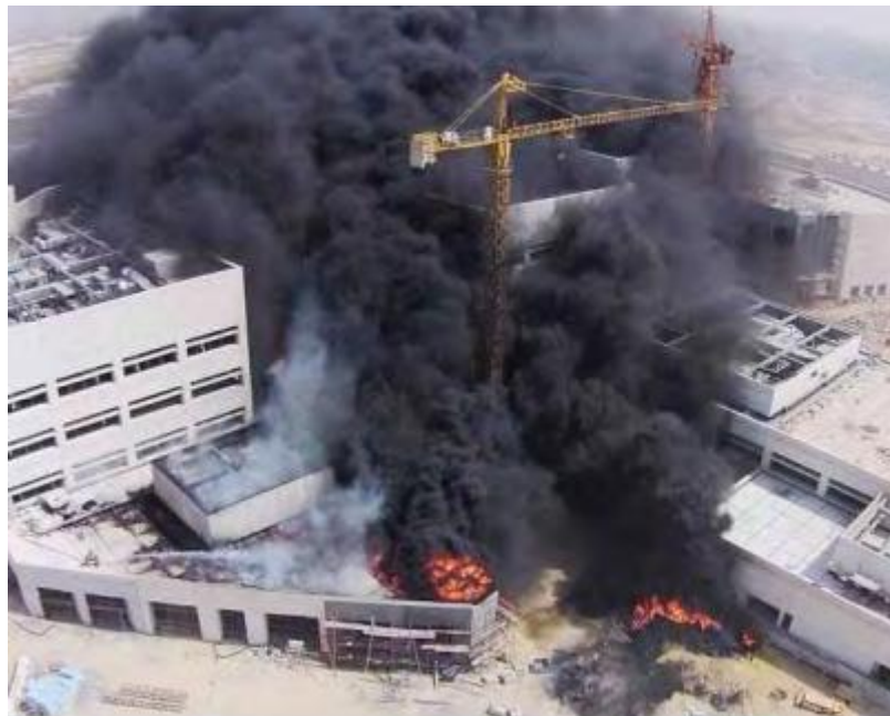
Figure 11: Outbreak of Fire at New KOC Hospital (26 th June, 2014)
